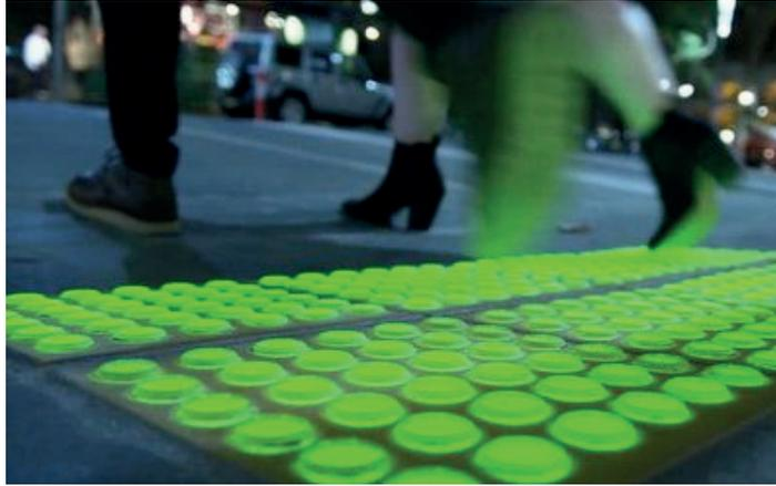
*Image Four, Melbourne In-Ground Traffic Light*
